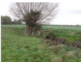
Looking north west at the bridge from the field
