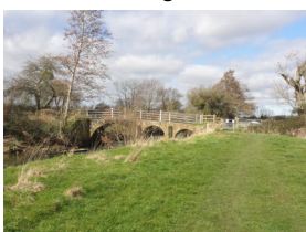
Looking north to the gate and bridge
