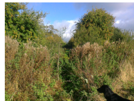
Looking north at the bridge from the field
